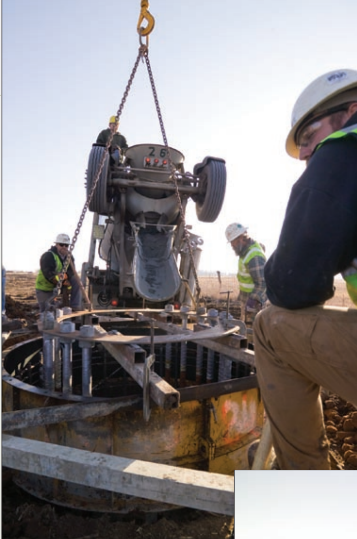
Contractors pour the concrete foundation for a steel pole for phase one of the 345 kV Wichita to Hutchinson to Salina line. Phase one extends from Wichita to Hutchinson. Phase two continues from Hutchinson to Salina.
