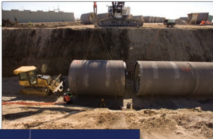
Construction on the circulating water line replacement on unit 3 at Jeffrey Energy Center.
