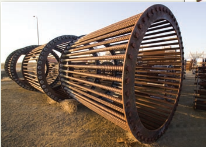
Contractors construct the 40 foot long rebar cages that will serve as part of the foundation for hundreds of steel poles.
