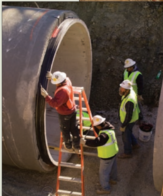
Crews prepare to seal a section of the new water line on unit 3.
