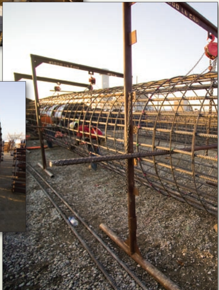
Contractors construct the 40 foot long rebar cages that will serve as part of the foundation for hundreds of steel poles.
