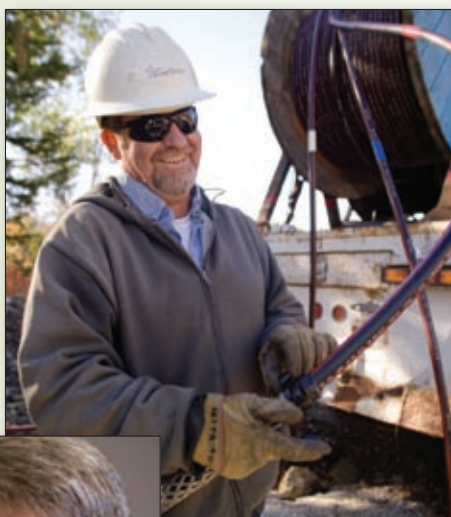
Craig Hansberry, Shawnee Division line foreman, prepares underground primary cable that will be used to service a new residential development.
