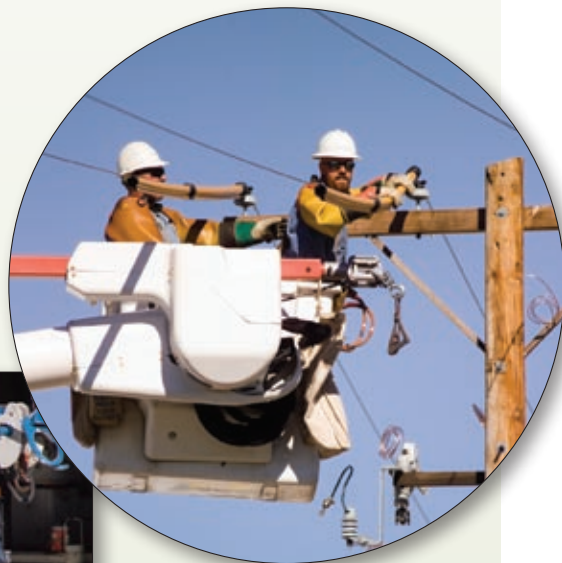
Ryan McCallister, apprentice lineman, and Robert Heath, journeyman lineman, install protective cover up on a line in preparation to provide service to a new commercial customer in DeSoto.
