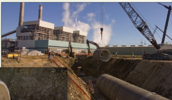
Construction on the circulating water line replacement on unit 3 at Jeffrey Energy Center.
